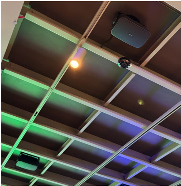
Sonance in-ceiling and surface mount loudspeakers cover the bulk of the venue.
