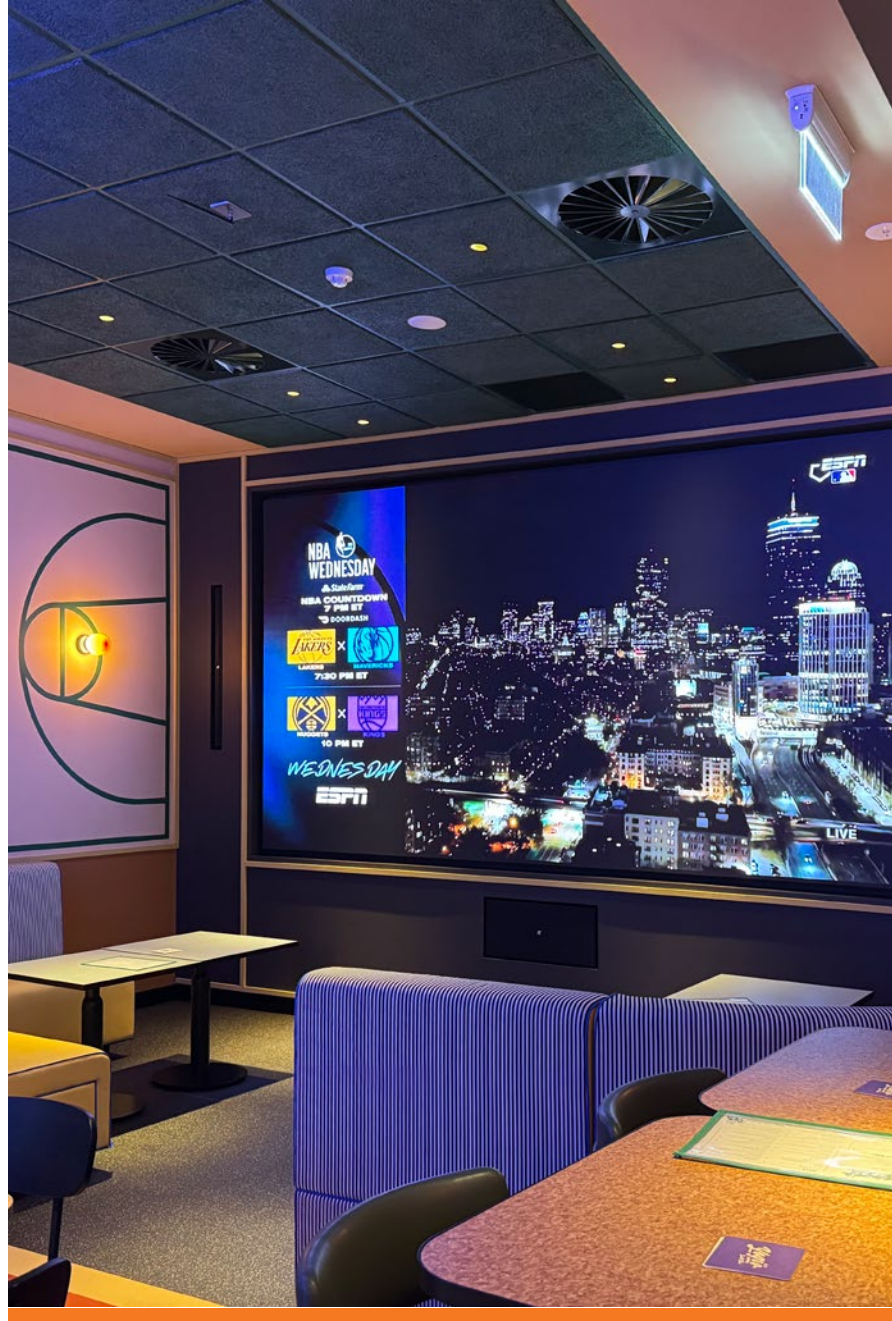
Sonance in-ceiling and surface mount loudspeakers cover the bulk of the venue.
