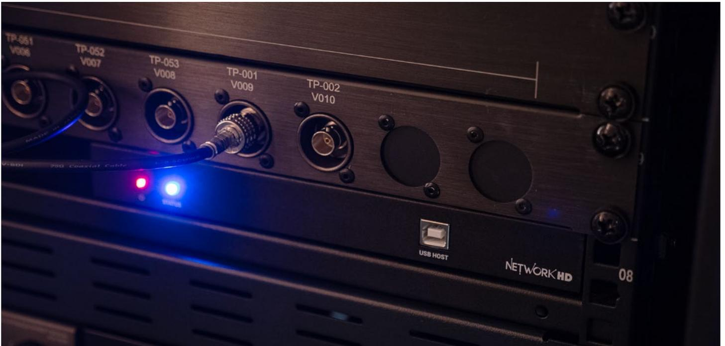
Multiple encoder endpoints take feeds from lectern HDMI inputs, the stage manager’s box, and the AVer PTZ camera (used primarily for stage replay). These sources can be distributed throughout the building, including to classrooms repurposed as dressing rooms during productions.
