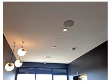
A total of nine (9) Apart ceiling speakers are also installed in the below hallway with the speakers above the timber slats. Some speakers have been sprayed black to hide them from view.
